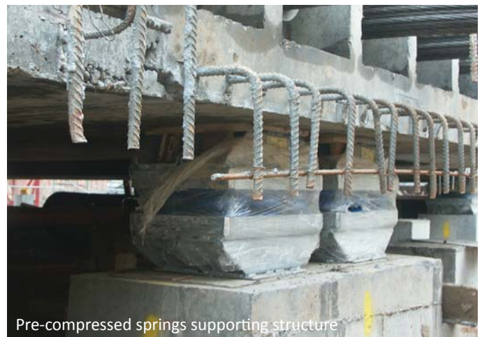
Pre-compressed spring boxes being placed on foundation
