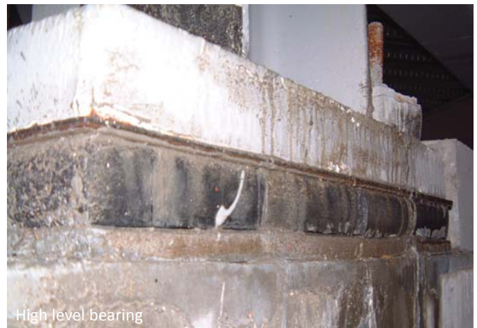
Bearing installed prior to grouting
