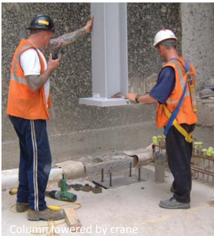
Column lowered on to bearing
