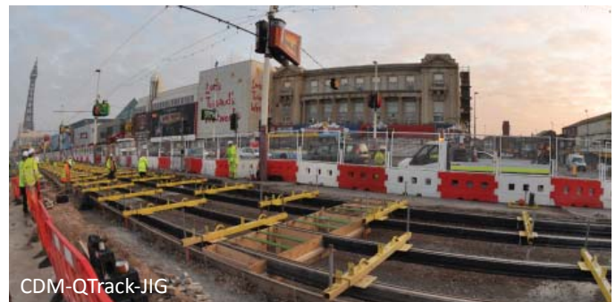
CDM-QTrack-JOG being installed January 2010
