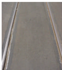
after the works
