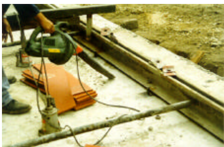
2. Pour concrete to underside of fixing
