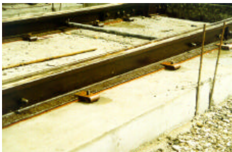
3. Install CDM-ISO-SRS railstrip beneath rail
