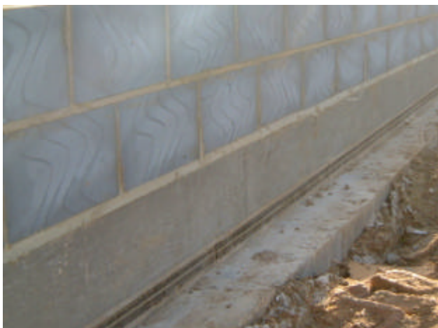
Load bearing masonry strip, 11Hz
