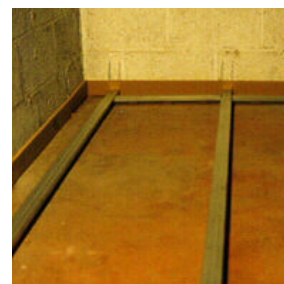
Installation of rails
