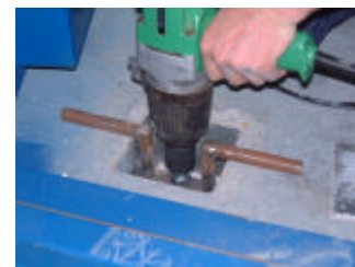
Jacking up the slab
