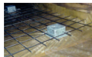
The boxes with reinforcement
