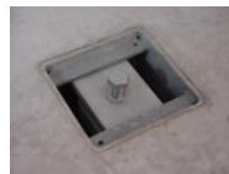
Ready for jacking
