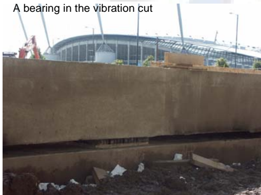
A bearing in the vibration cut
