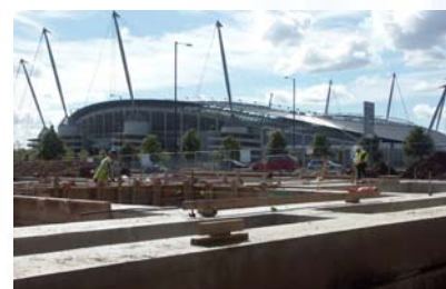
3 no. bearings grouted to the top of the ground beam
