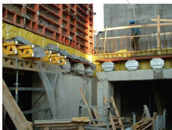
Installation on site
