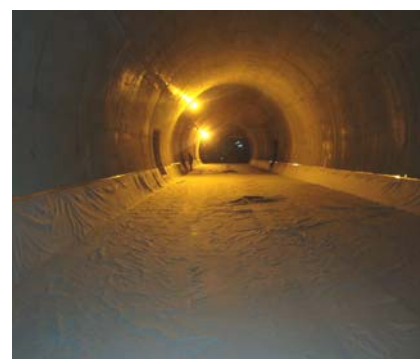
Metro tunnel Lisboa
