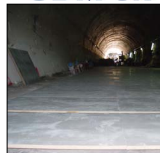
The installation of the panels
