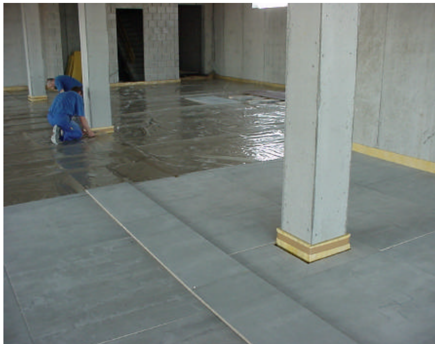
Installation of the PVC waterproof membrane
