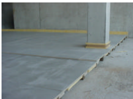
Installation of the panels
