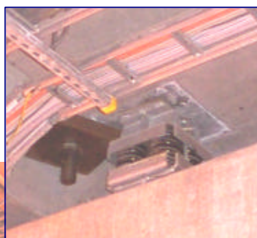
Detail of CDM-CHR-B4 springbox on top of RC beam structure
