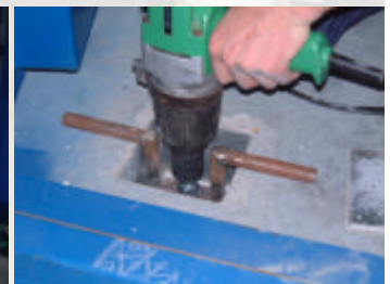
Jacking the slab up
