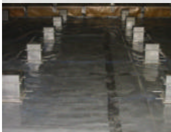
The installed jacks
