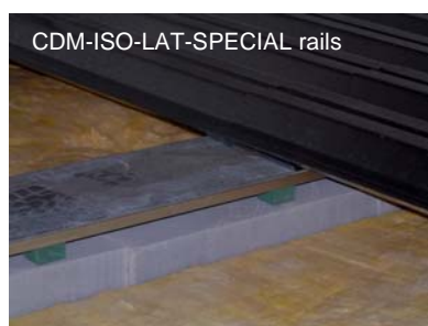
The rails with decking
